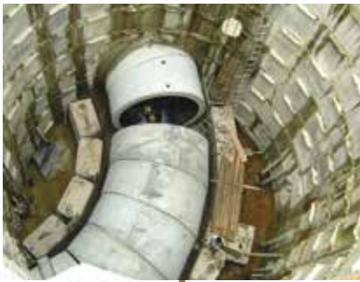
PUB Deep Tunnel Sewerage System
