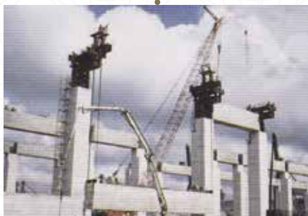
PSA Overhead Gantry Structure Phase 1A
