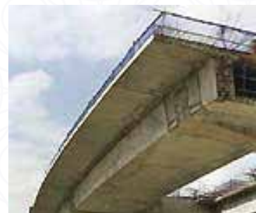
Upper Serangoon Viaduct
