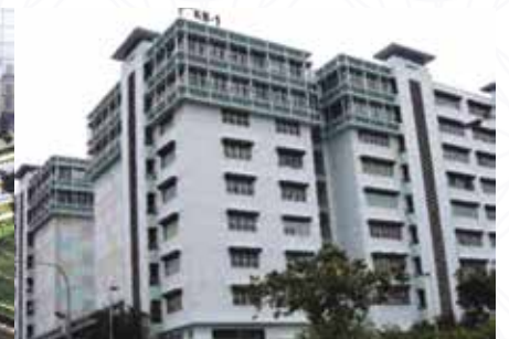
Jurong Town Corporation Factory at Kaki Bukit - Phase 2
