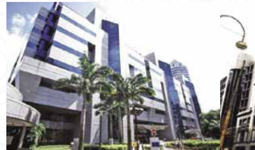
Alexandra Technopark Warehouse Blk A at Alexandra Point
