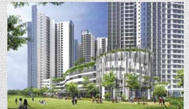
HDB Housing Development at Kallang Whampoa
