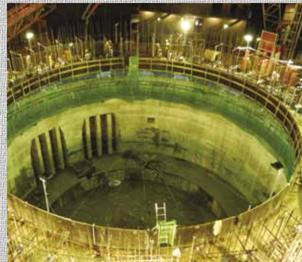
Construction of 25,000 Tonne Cement Silo
