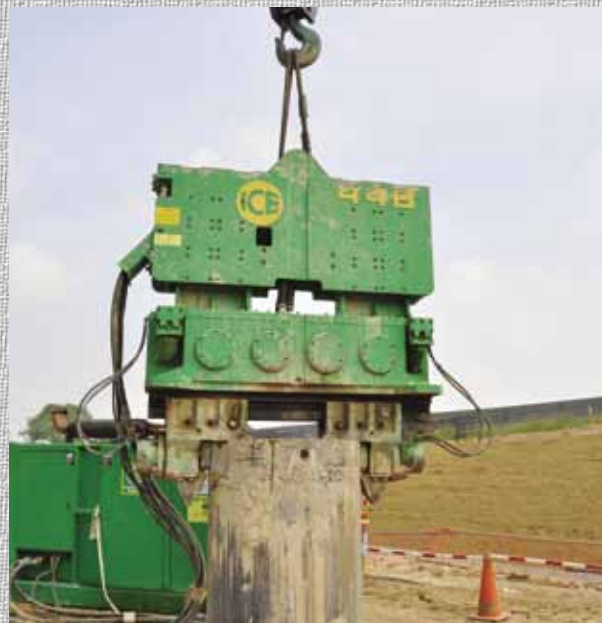
Bored Pile Casing Extraction
