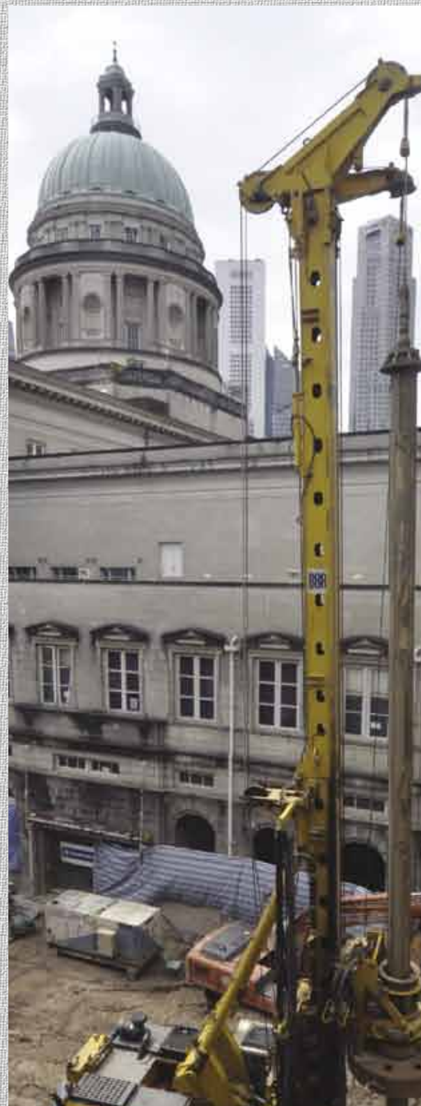
Bored Piling Work at National Art Gallery
