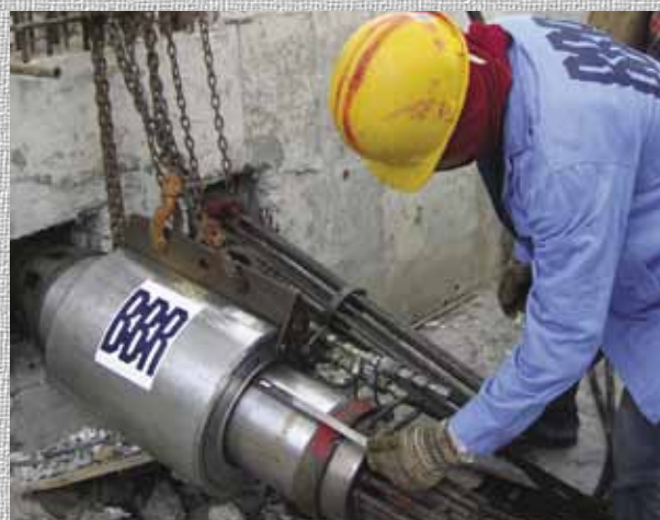
Post-tensioning Work
