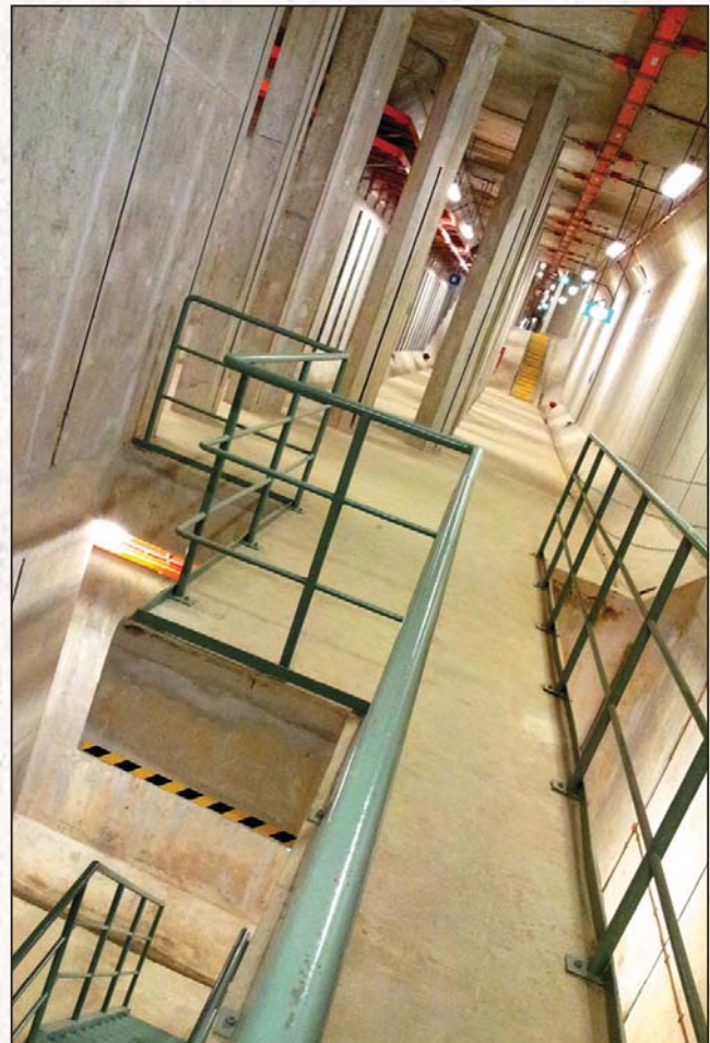
Common Services Tunnel Phase 3A in Marina Bay, Singapore
