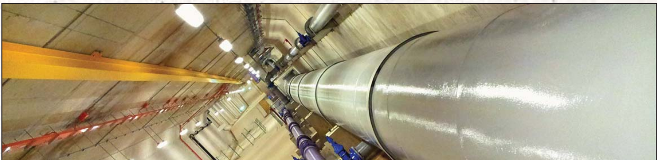
Common Services Tunnel Phase 3A in Marina Bay, Singapore
