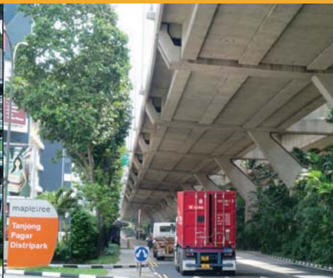
2] Keppel Viaduct, Singapore
