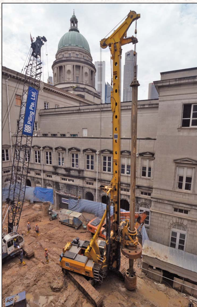
Bored piling works
