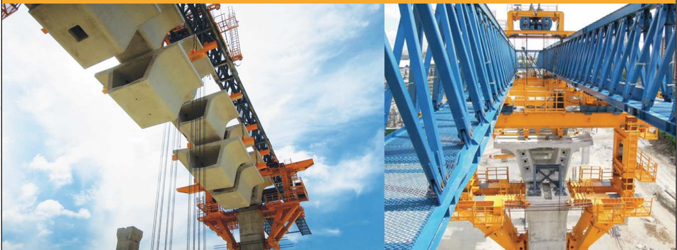
7] Kelana Jaya LRT Line Extension Project in Malaysia
