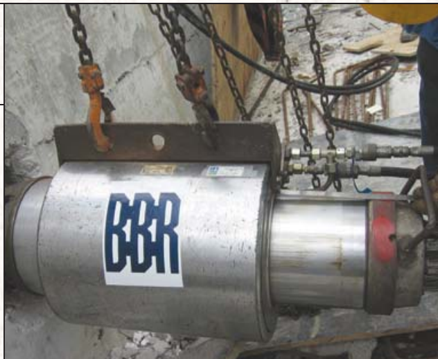
Prestressing in progress
