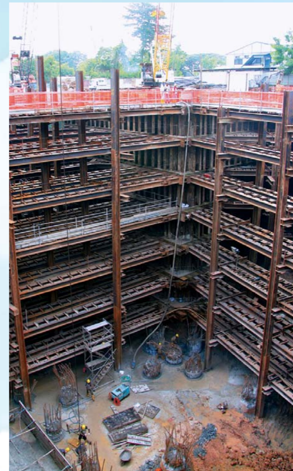
Common Services Tunnel Phase 3A @ Downtown Core
