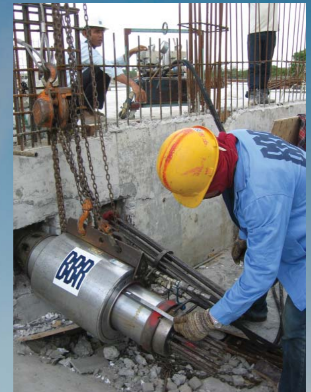
Prestressing in progress
