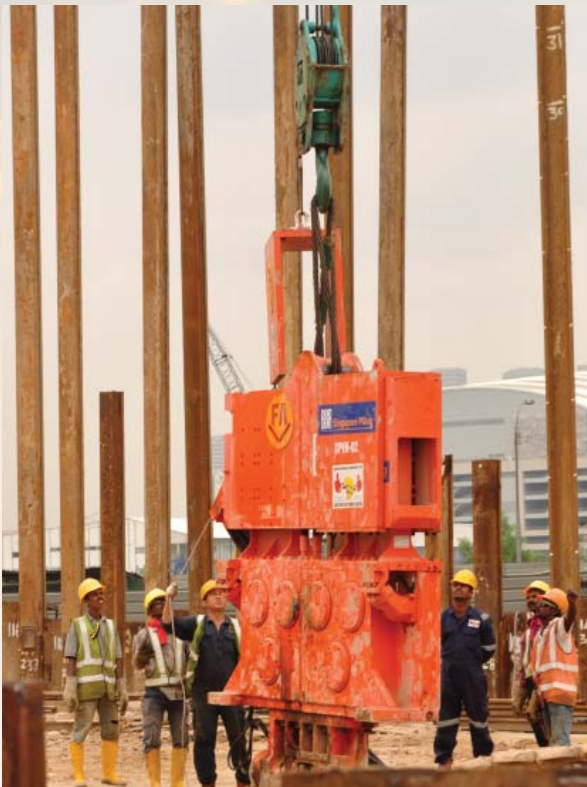
Common Services Tunnel Phase 3B @ Downtown Marina Bay
