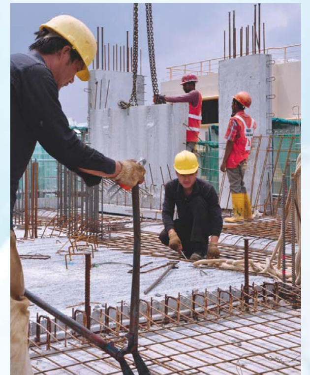
Construction work @ Yishun HDB
