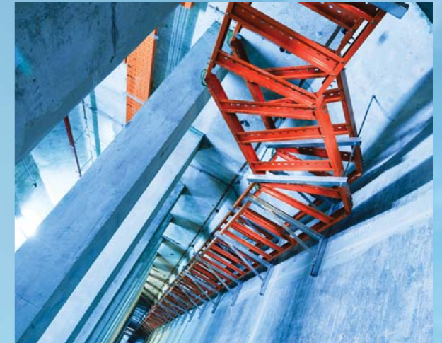
Common Services Tunnel Phase 3A @ Downtown Core
