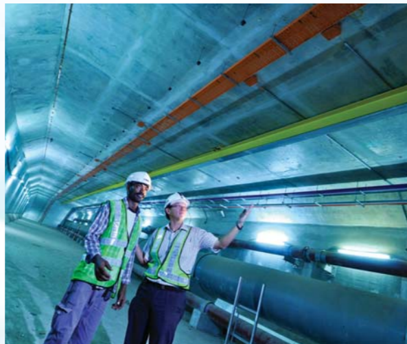
Common Services Tunnel Phase 3A @ Downtown Core
