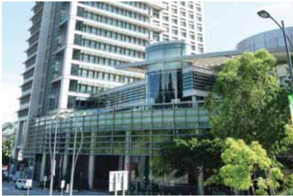
Ministry of Education (MOE) HQ Building (Post-tensioning)
