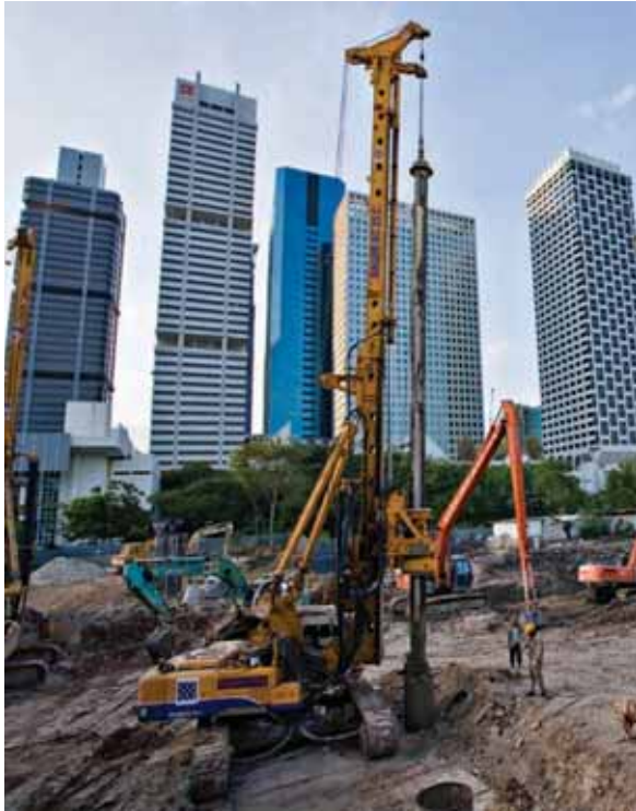
Common Services Tunnel (CST) Phase 3A @ Marina Bay
