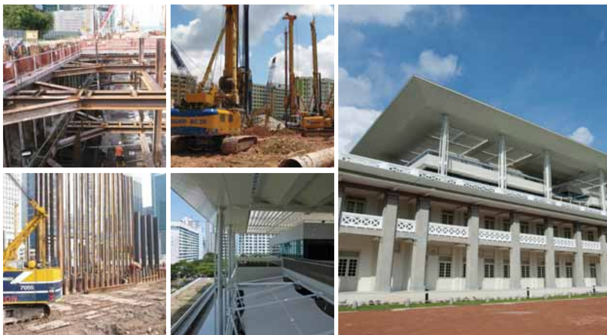
Common Services Tunnel (CST) Phase 3A @ Marina Bay
