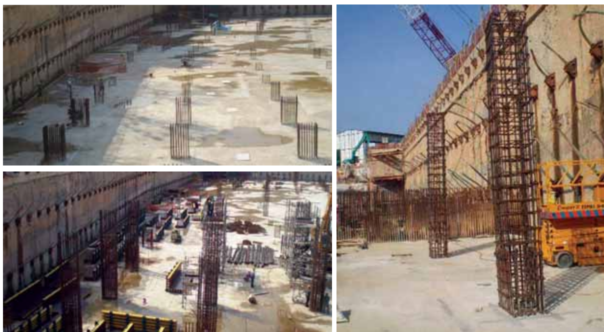
Khoo Teck Puat Hospital (Basement Construction)
