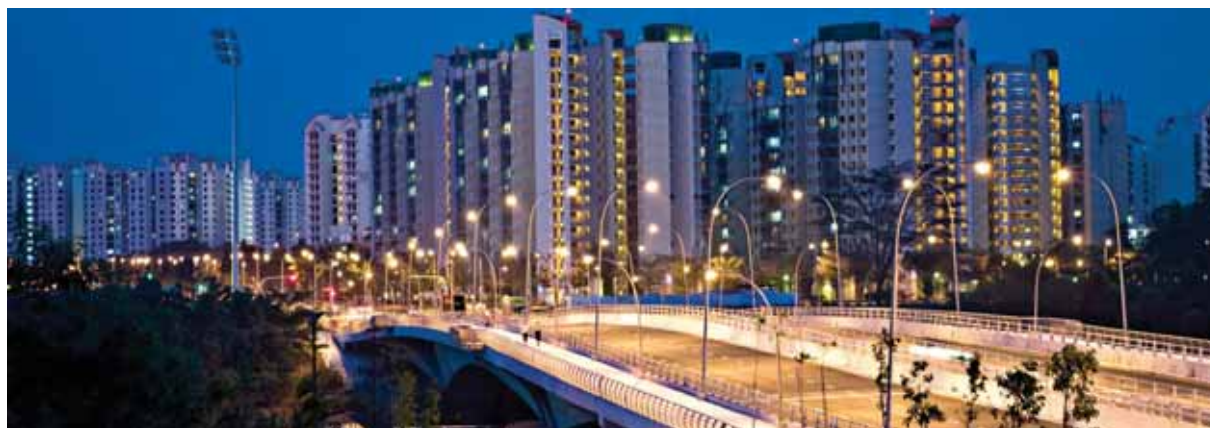
Middle Bridge across Sungei Punggol
