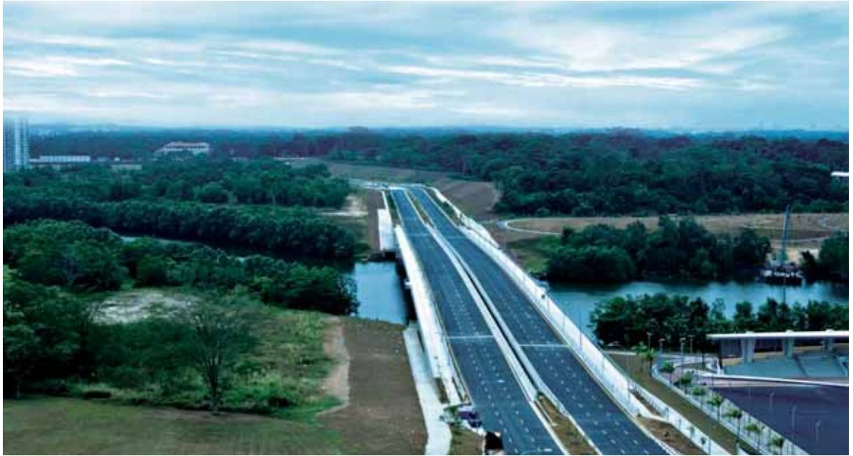
Middle Bridge across Sungei Punggol
