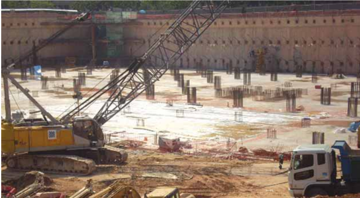
Khoo Teck Puat Hospital (Basement Construction)
